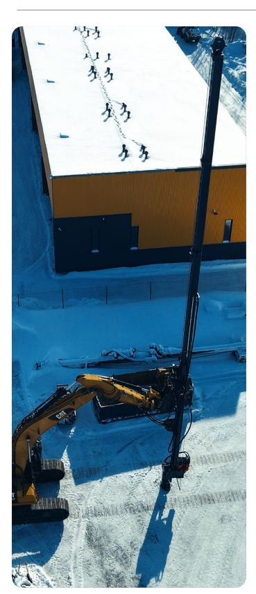
MOVAX column stabilisation leaders provide a versatile solution for column stabilisation utilising both dry and wet binder material.
