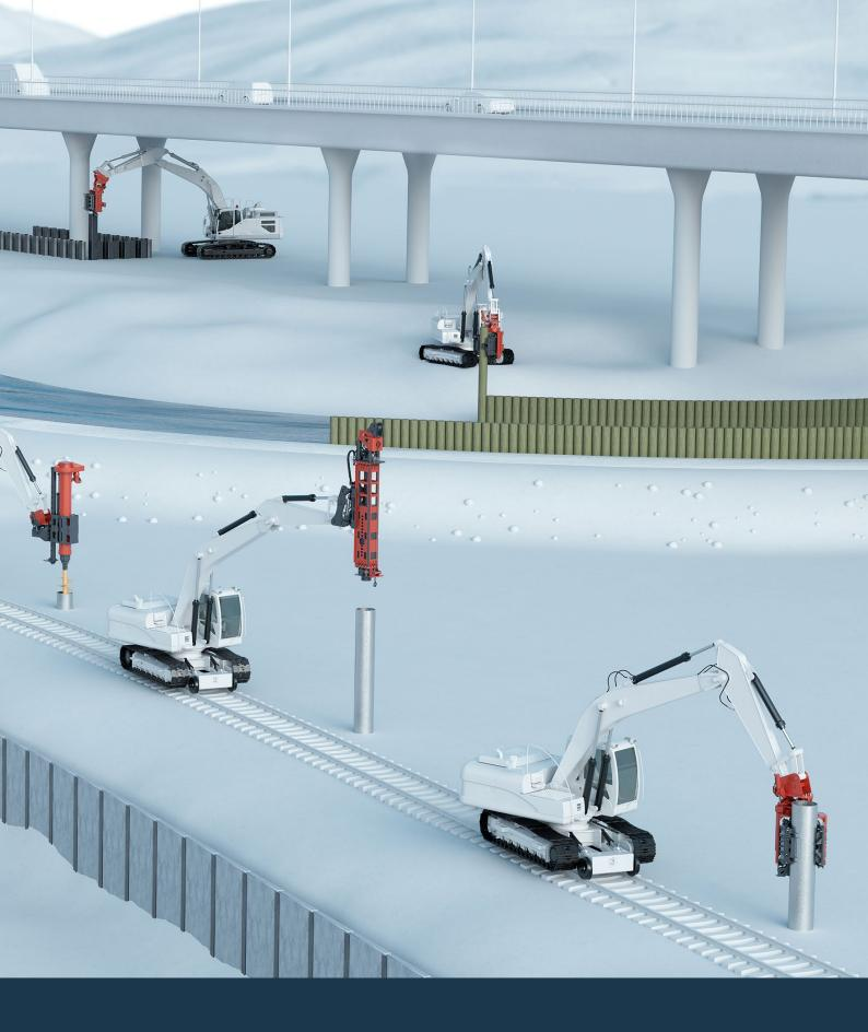
MOVAX WAY-OF-PILING™ provides the optimum way of working when constructing load bearing foundations, building retaining walls, both temporary and permanent, cofferdams and when performing trenching and excavation work; and soil stabilisation in a wide range of applications.
